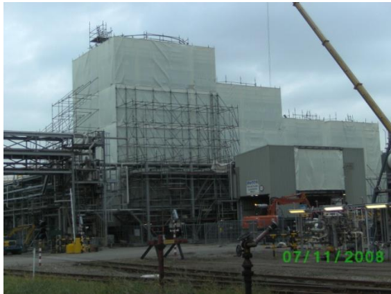
Above is the Encapsulation around Tanks
