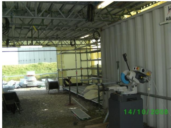
Above is a Temporary Workshop
